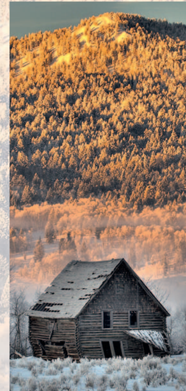
(a) This lonely, decaying cabin, though badly twisted and bent, continues to hold out against Idaho's brutal mountain winters. The dynamic range between the sunlit snow on the mountain and the shaded wood under the roof is far too wide to be successfully recorded in a single image. Five images were shot to fully capture the dynamic range. These included the standard exposure, +2, +4, -2, and -4 stops of light. These images were merged into one single tone-mapped image using Photomatix Pro. Final image adjustments were done with Photoshop CS3.
